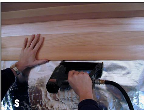
**16.** Continue fastening your T&G along the wall (figure S) till you reach your last board either at the top or bottom. You may need to rip your last board to fit making sure your bottom board is at least 1/4" off the floor. Finish the rest of the interior in the order of back wall, side walls, and lastly the front (door) wall.
